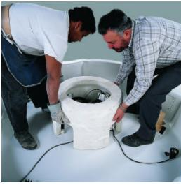
ting from the end of the unconnected pump hose and put aside for use in Step 10. Note, the connections for alternate Center Pieces vary slightly for each Center Piece; consult the instruction specific to your Center Piece in Appendix A, Step 11A.
